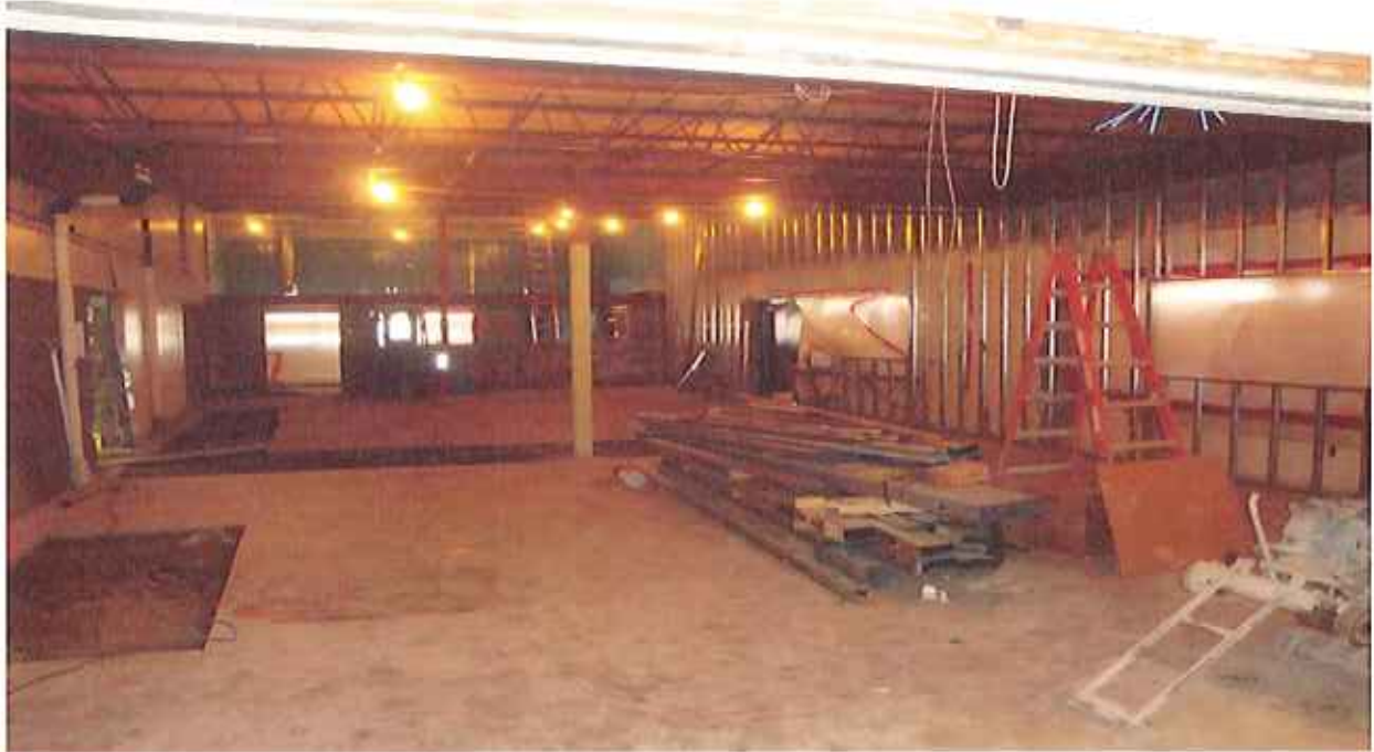
Main CTE Building – PHASE J: HORTICULTURE SHOP – NOVEMBER 2013
