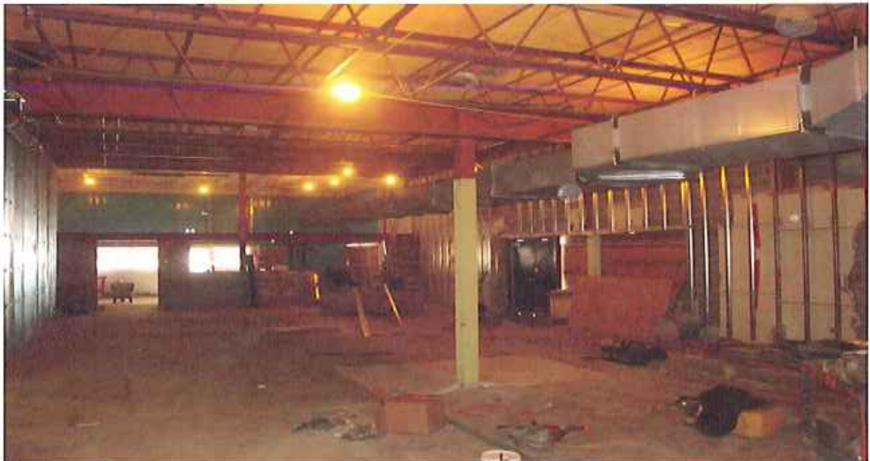
Main CTE Building – PHASE J: HORTICULTURE SHOP – DECEMBER 2013
