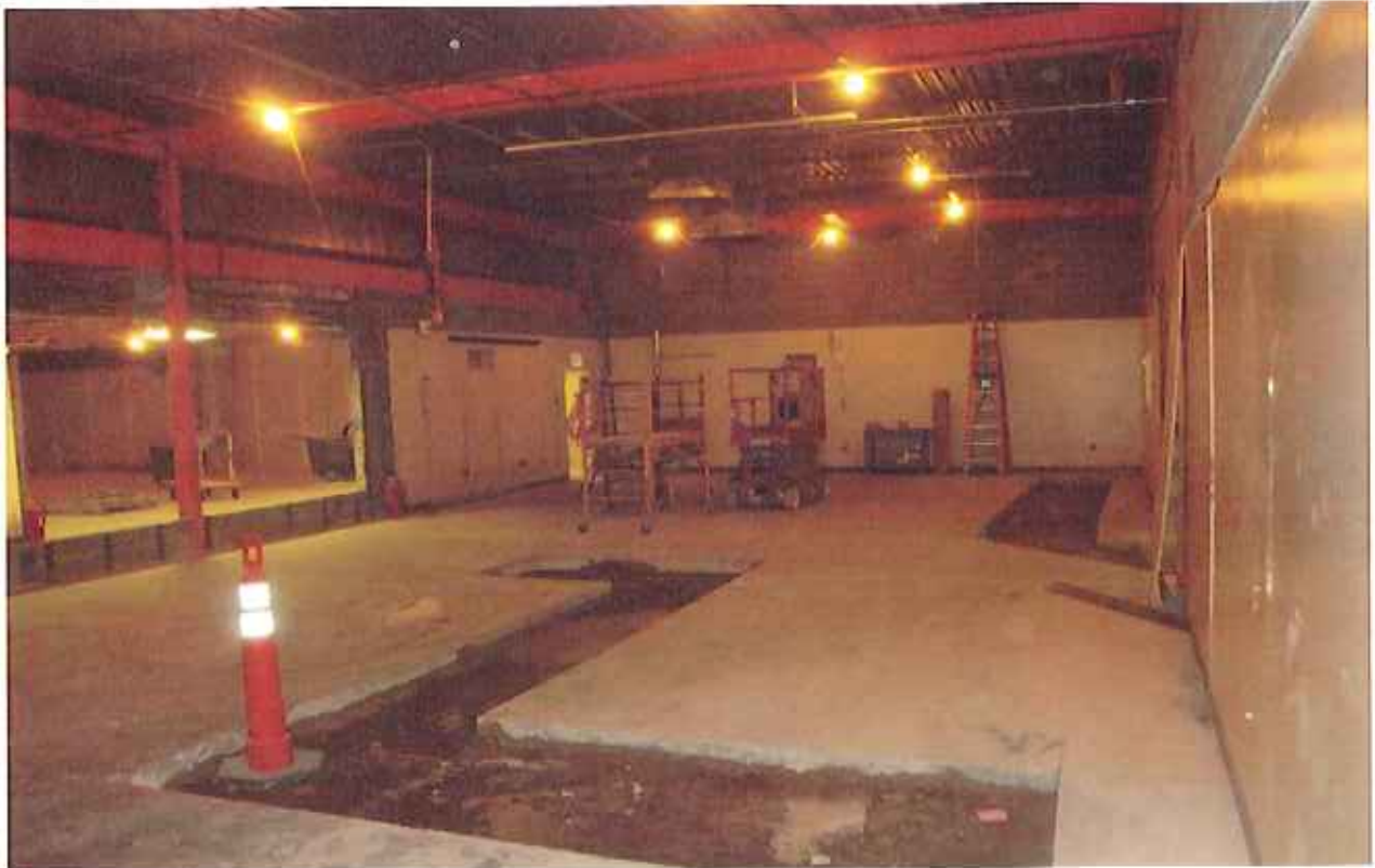
Main CTE Building – Phase K: Computer Technology – November 2013
