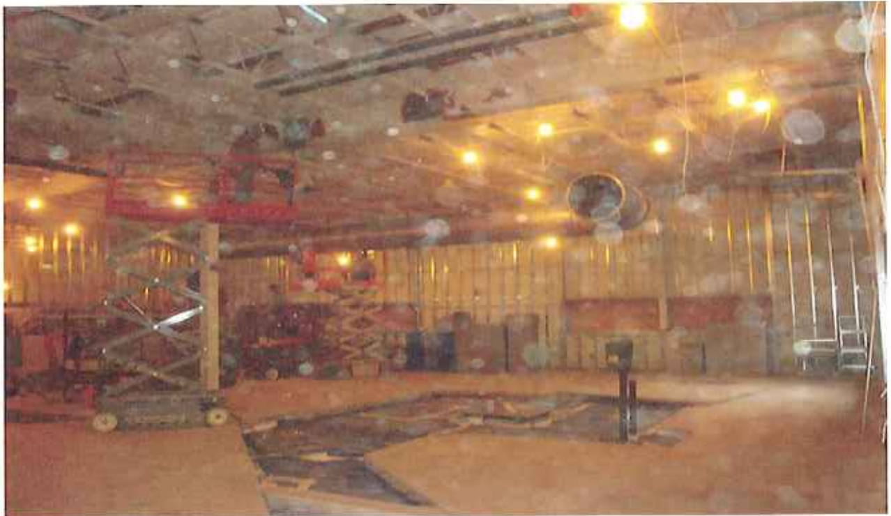
Trades Building – Phase Q: Outdoor Power Shop – November 2013
