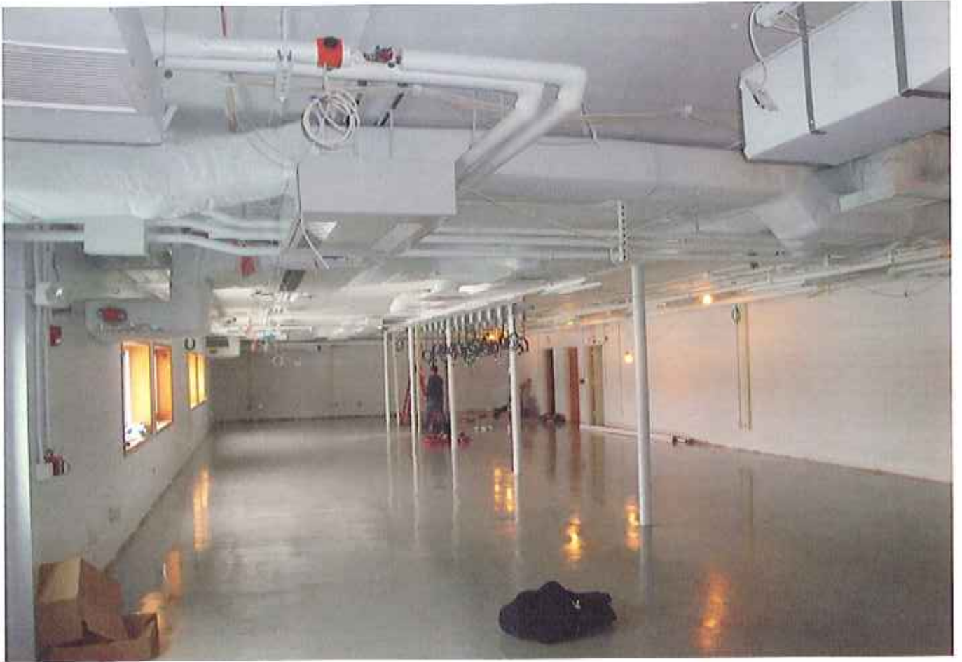
BUILDING B – NEW PRINT SHOP – DECEMBER 2013
