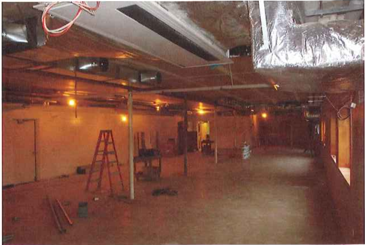
W450 – Phase U: New Print Shop Renovation. Demolition Completed. Mechanical Rough-In and Ceiling / Wall Patch and Prep for painting ongoing.
