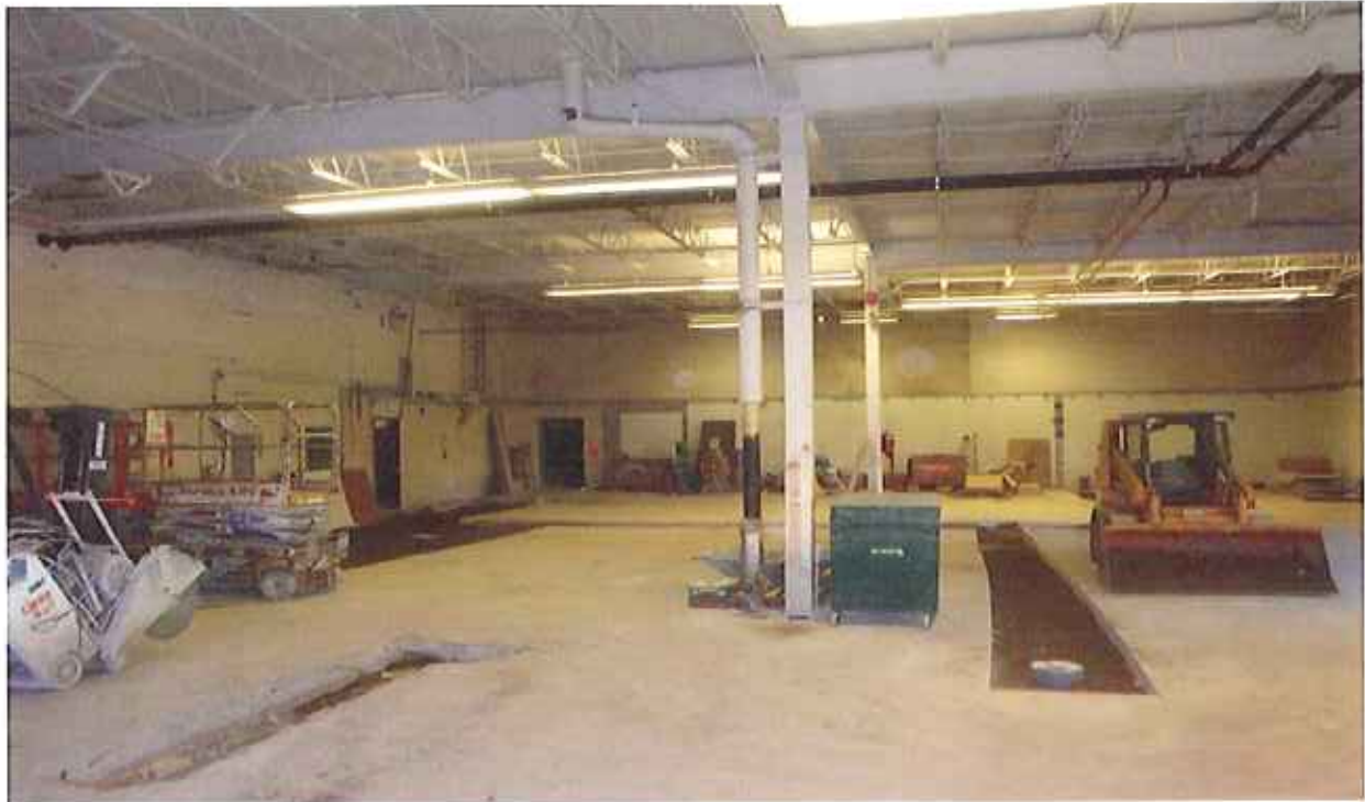
Trades Building – Phase P: New Construction Tech Shop. Demolition Complete, underground sanitary rough-in complete, overhead mechanical rough-in started.
