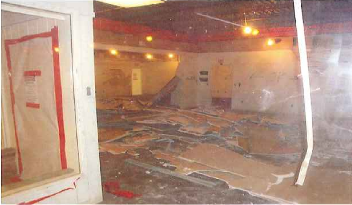
Main CTE Building – Phase H: Wall Demolition, ACM Mastlic Discovery.
